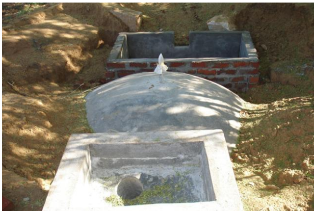
Constructed Deenabandhu Biogas Unit
