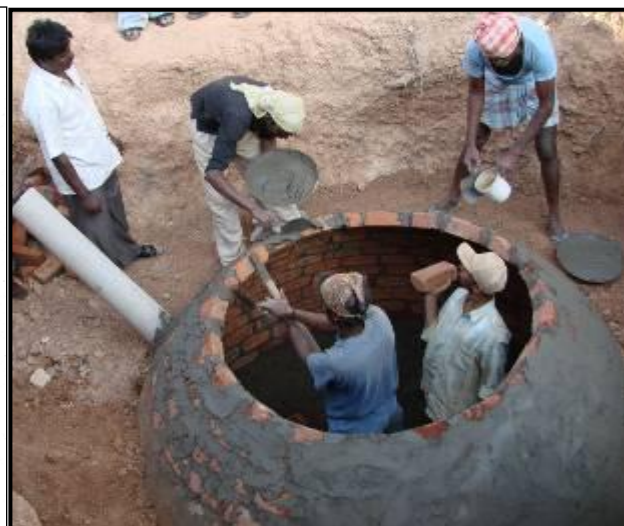
Construction of Biogas Plant
