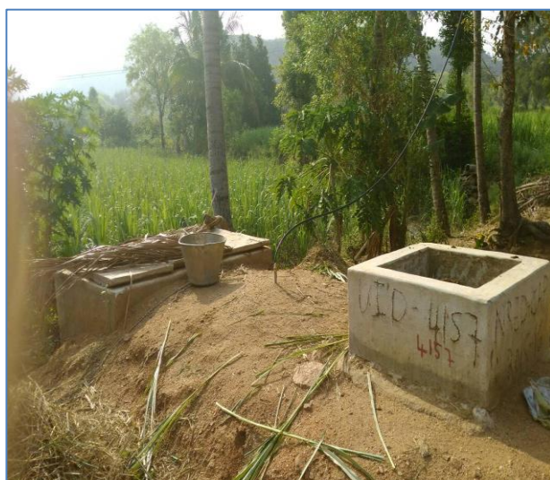
Deenabandhu Model Biodigester
