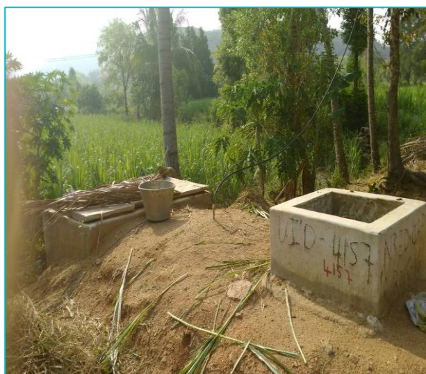
Deenabandhu Model Biodigester
