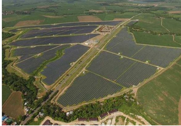
Figure 2. Location of Manapla 48MW Solar Power Plant
