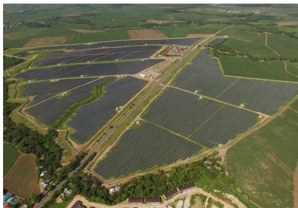
Figure 2. Location of Manapla 48MW Solar Power Plant
