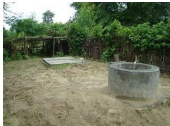
Fig 2: Biogas Digester in Operation
