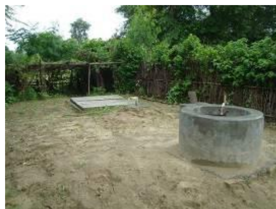
Fig 2: Biogas Digester in Operation
