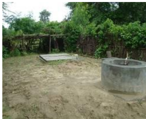
Fig 2: Biogas Digester in Operation
