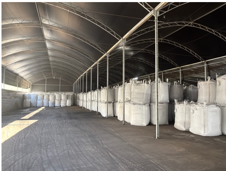
FIGURE 6: BIOCHAR STORAGE AREA
