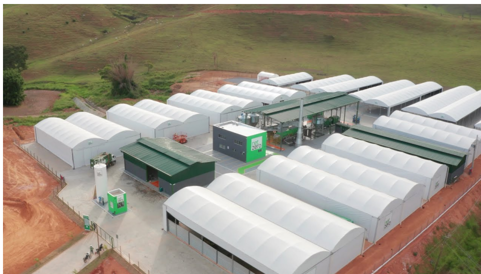
FIGURE 1: NETZERO LAJINHA FACILITY
