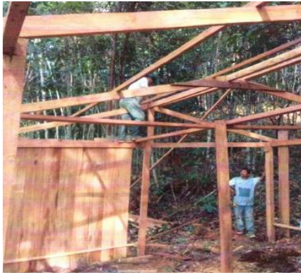
Illustration 23. Construction in Sector 3a
