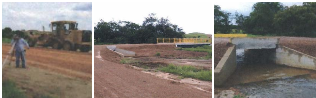
Illustration 45. Improvements made in the road from Cumaribo towards Cumariana
