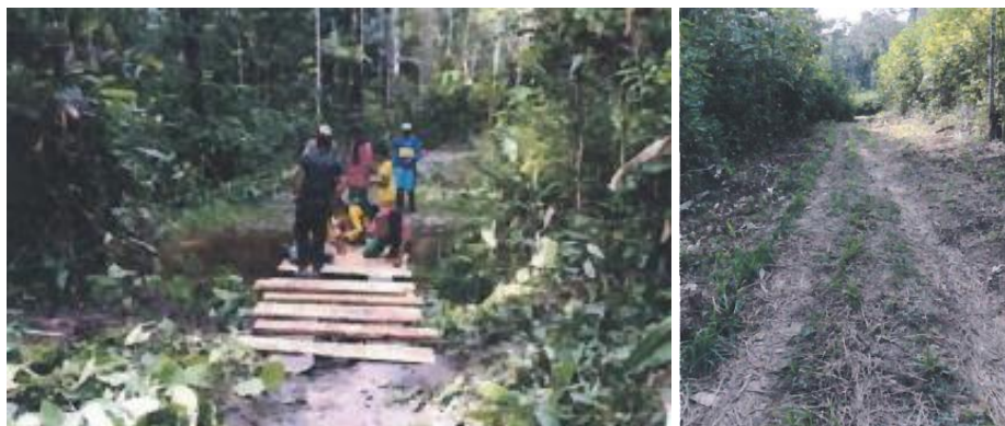
Illustration 41. Pedestrian bridge in Kirey Central and maintenance in road towards Corocito
