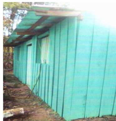
Illustration 22. Control station in Sector 2
