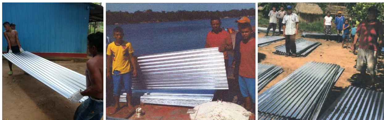
Illustration 97. Sheets of zinc to improve the quality of roofs in homes in RIU-SM
