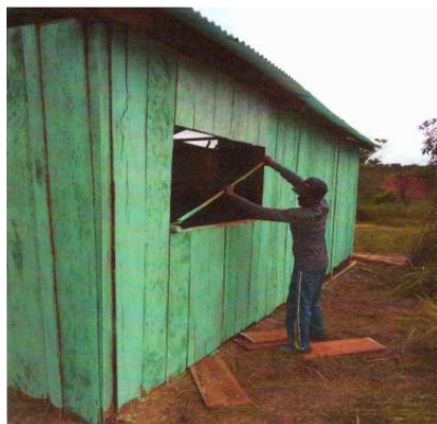
Illustration 21. Control station in Sector 1
