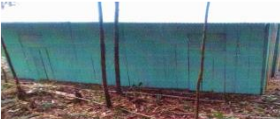
Illustration 25. Control station in Sector 4
