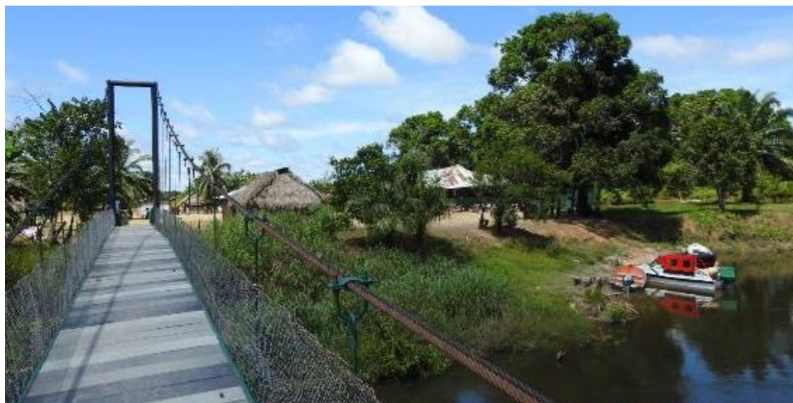
Bridge built with indigenous labor (Urba Morichal community, Zone 2 Bajo Río Vichada)
