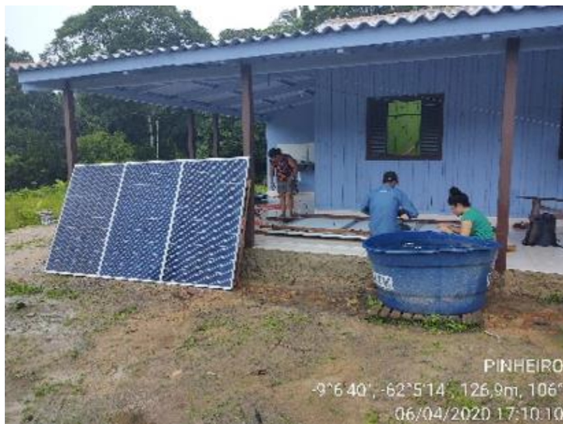
Figure 11 - Installation of the solar power kit in April 2020.
