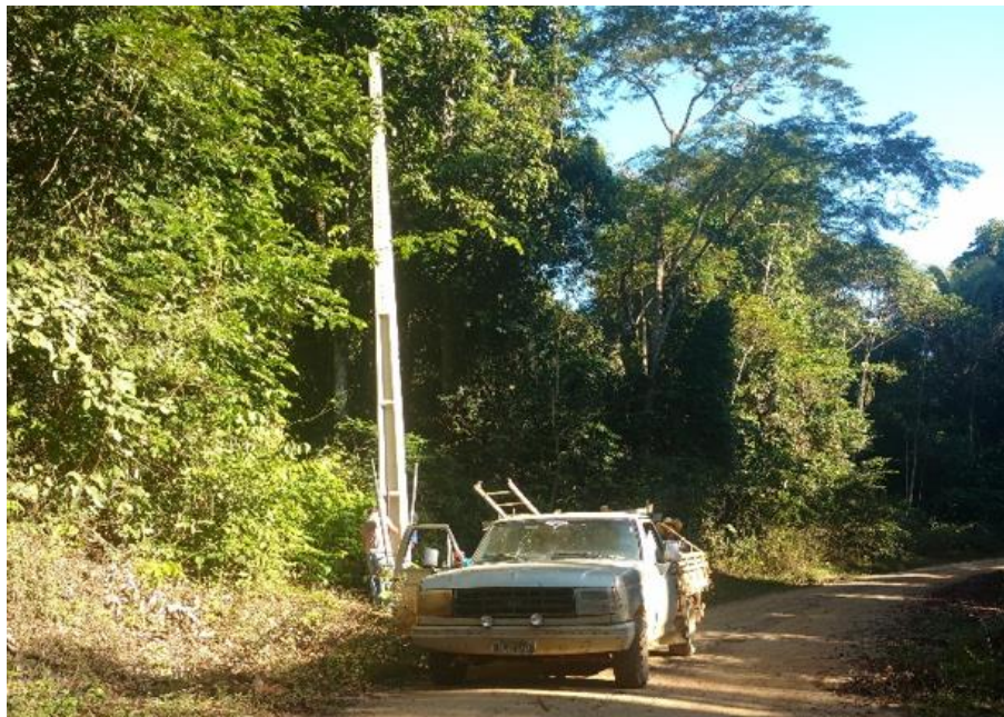
Figure 10 - Electrical network installation at RESEX Rio Preto-Jacundá.
