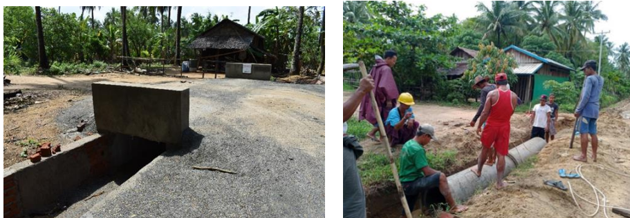
Figure 6: Construction of box culverts
