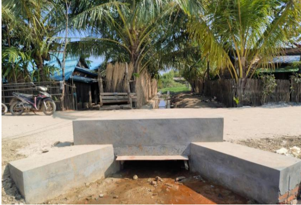
Photo 7: Box culvert and drainage construction at Shwe Thaug Yan Ward 3
