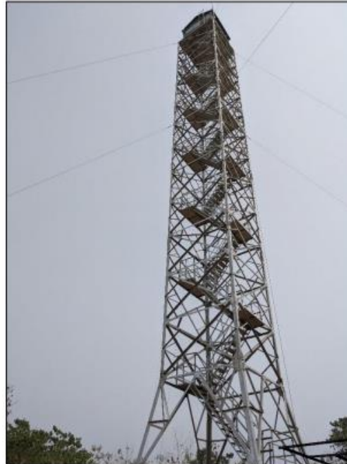
Photo 1-21: A fire watchtower with good sight lines of much of the plantation represents a significant investment in fire prevention. The site also houses a radio repeater providing coverage of the northern parts of the plantation.
