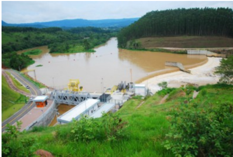
Figure 1 – Salto Pilão Hydropower Plant (source: CESAP’s website)
