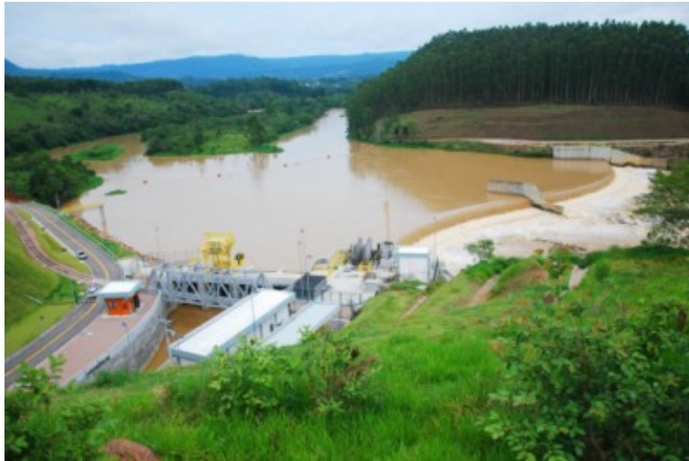
Figure 1 – Salto Pilão Hydropower Plant
