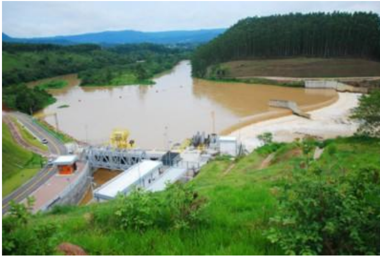
Figure 1 – Salto Pilão Hydropower Plant
