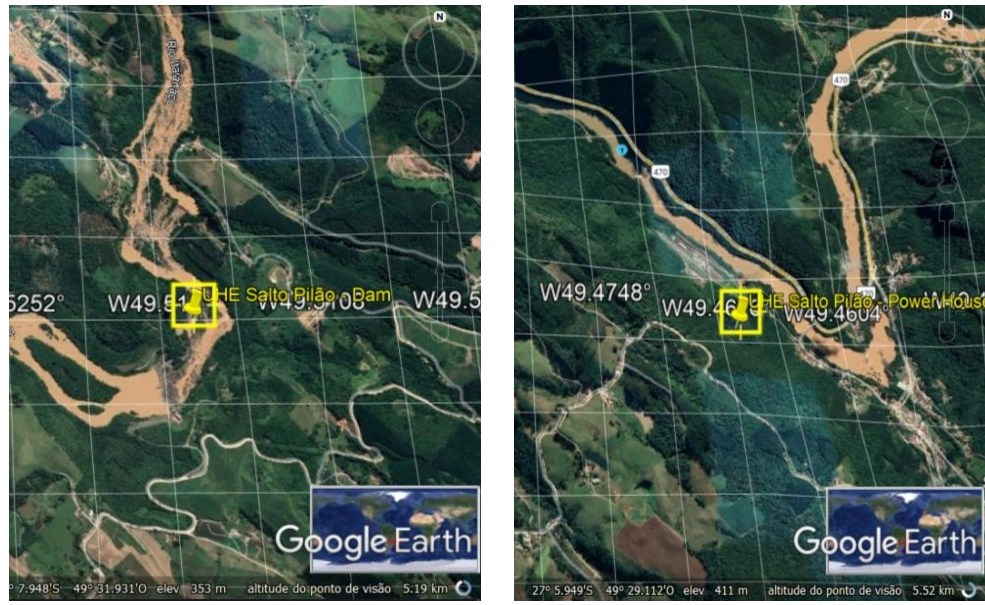
Figure 4 - Physical location of the Dam (left) and the Power House (right).
