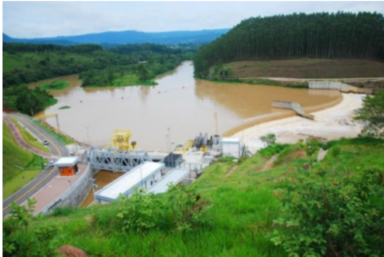
Figure 1 – Salto Pilão Hydropower Plant (source: CESAP’s website)
