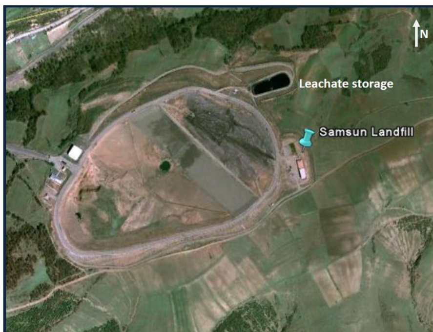
Figure 3. Current landfill site and the Project's location (at the eastern side)
