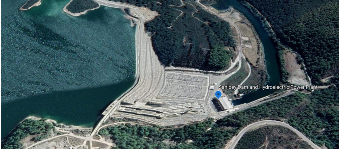
Figure 1: Satellite image of the Project
