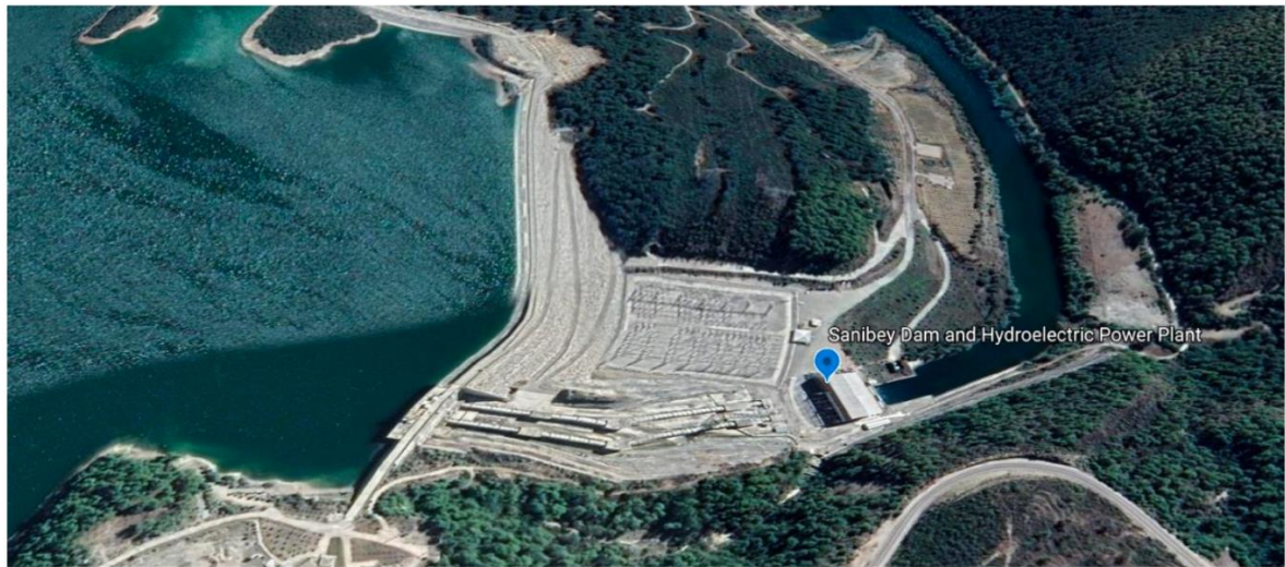
Figure 1: Satellite image of the Project
