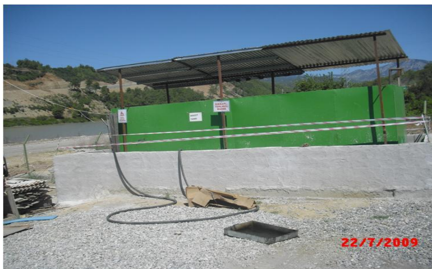
Figure 7: A scene of the storage of waste lubricants temporarily stored in closed containers located on an impervious platform at the construction site.
