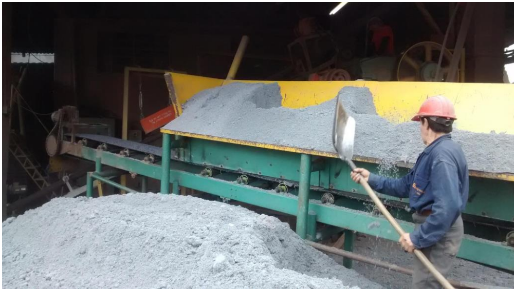
Figure 3. Employee loading pulp and paper sludge inside the molding machine
