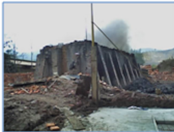
Figure 3. Pampa kiln at Santander Ceramic (pre-project situation).
