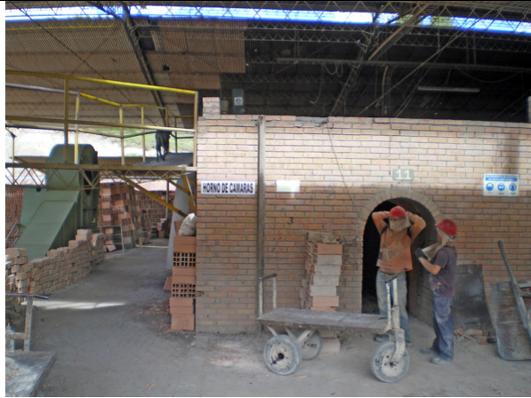
Figure 4. Chamber kiln at Santander Ceramic (project situation).
