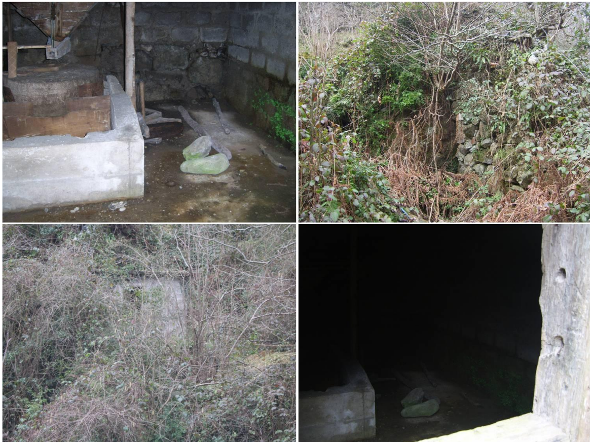
Figure 3. Corn mill in the diverted section of the river.
