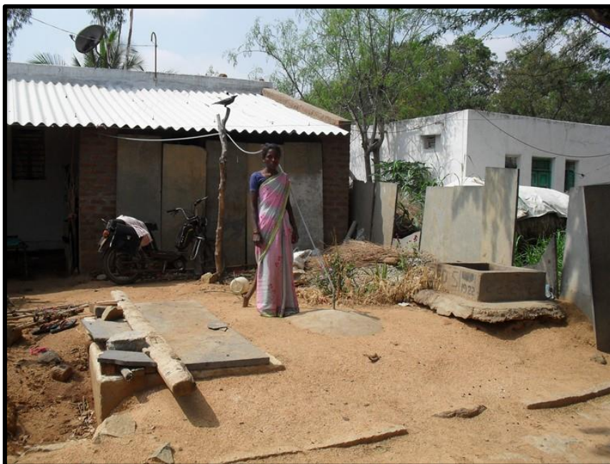
Figure 3: Biogas Unit with clean surroundings
