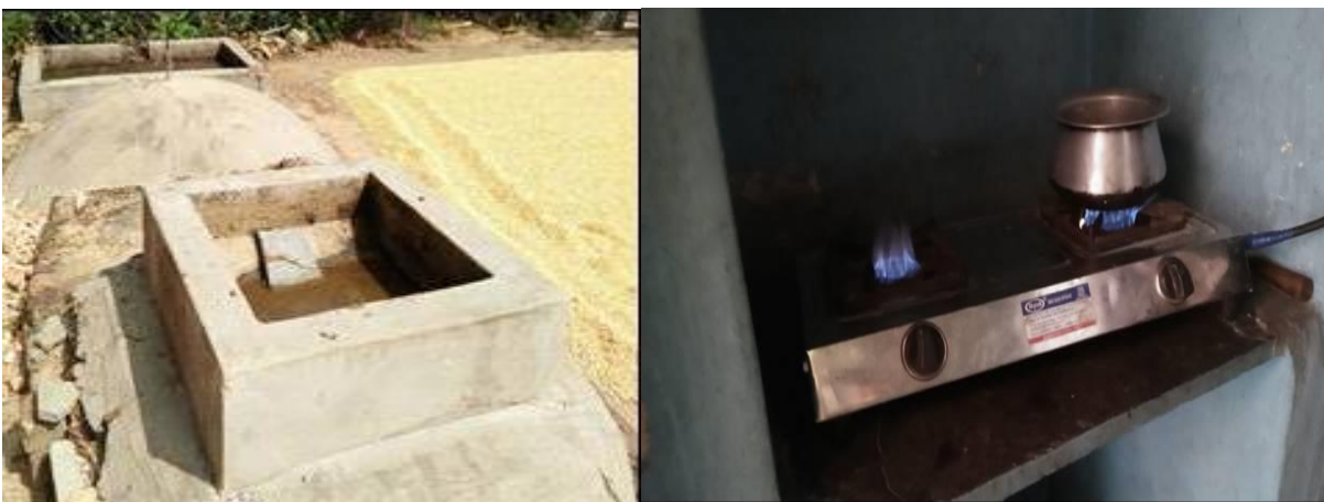
Fig 4: Constructed Deenabandhu Biogas Unit and Biogas Stove in the kitchen
