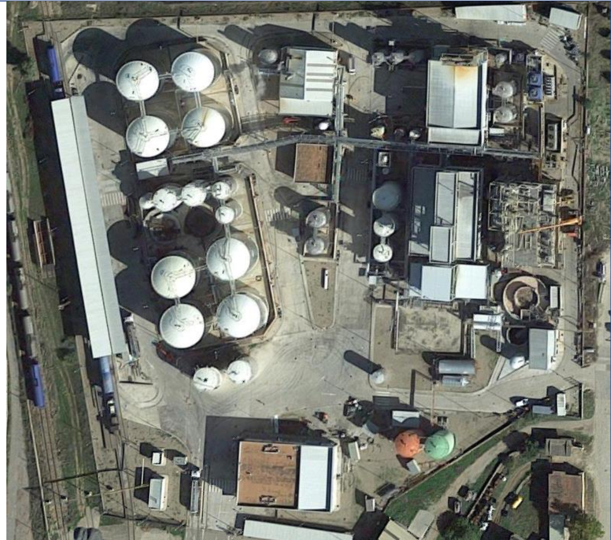
Figure 1. Aerial image of the plant.
