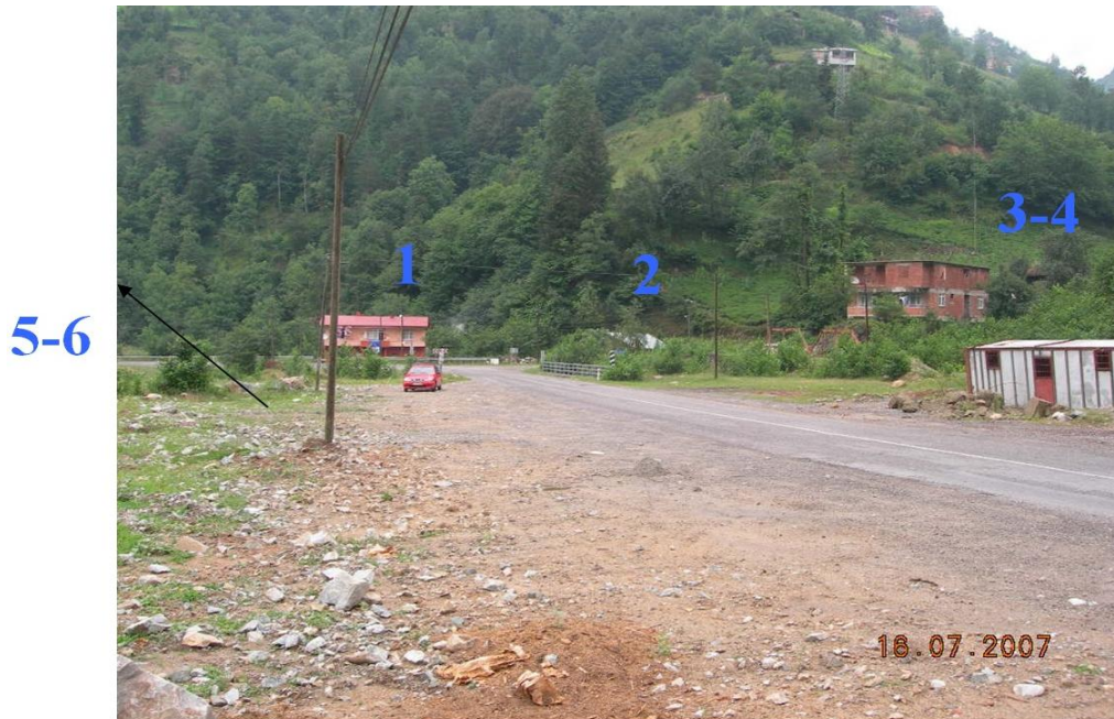
Figure 13: General view of weir site
