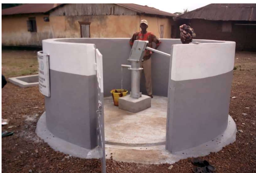
Left image: India Mark 2 pump in action from the project in Sierra Leone (Source: CO2balance)
