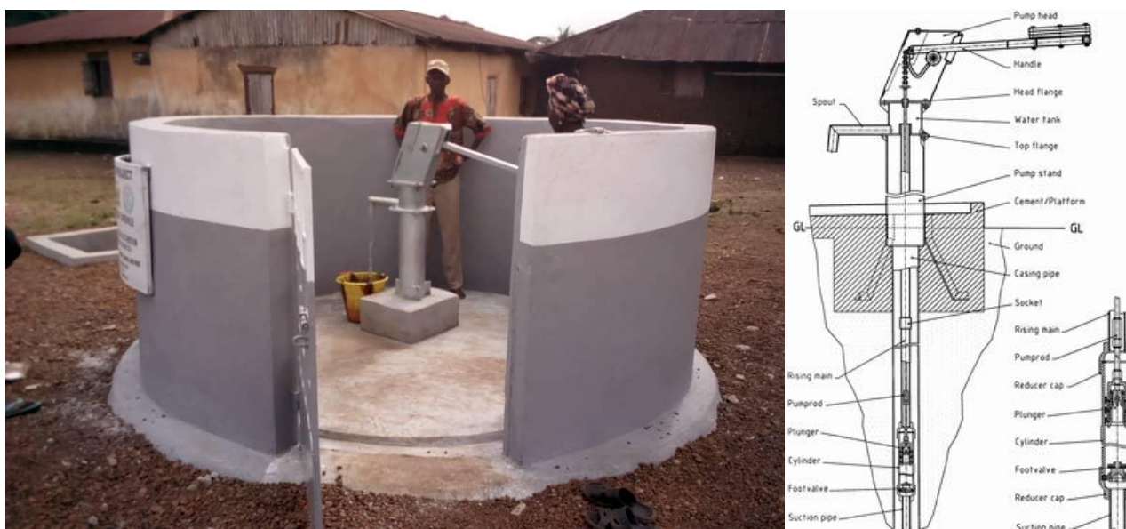
Left image: India Mark 2 pump in action from the project in Sierra Leone (Source: CO2balance)
