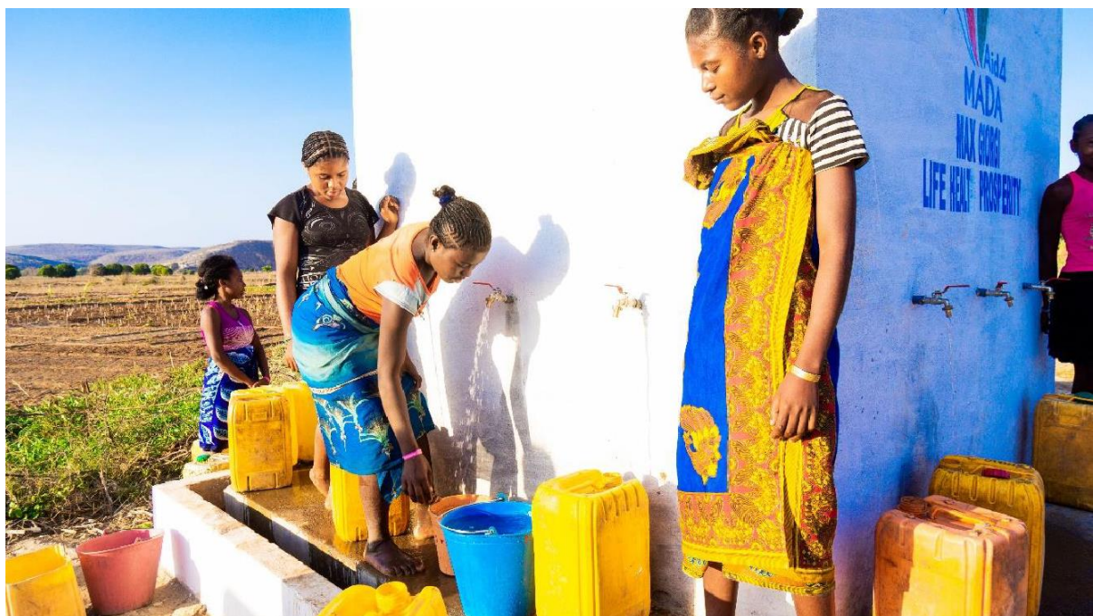
Imagines A-11. Project water system constructed in Mandrosoa village (GS10783)
