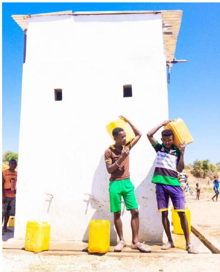
Imagines A-15. Project water system constructed in Maromiandra Antevamena
