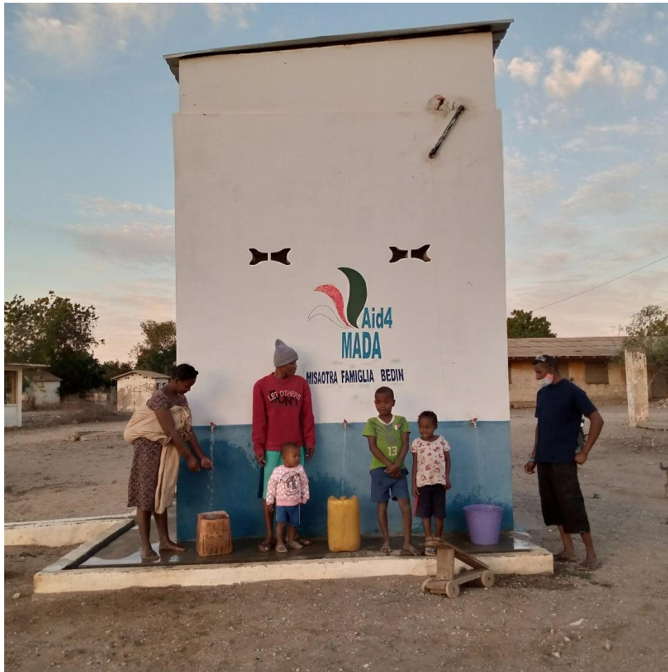
Imagine A-1. Project water system constructed in Belembohy Androvakely village
