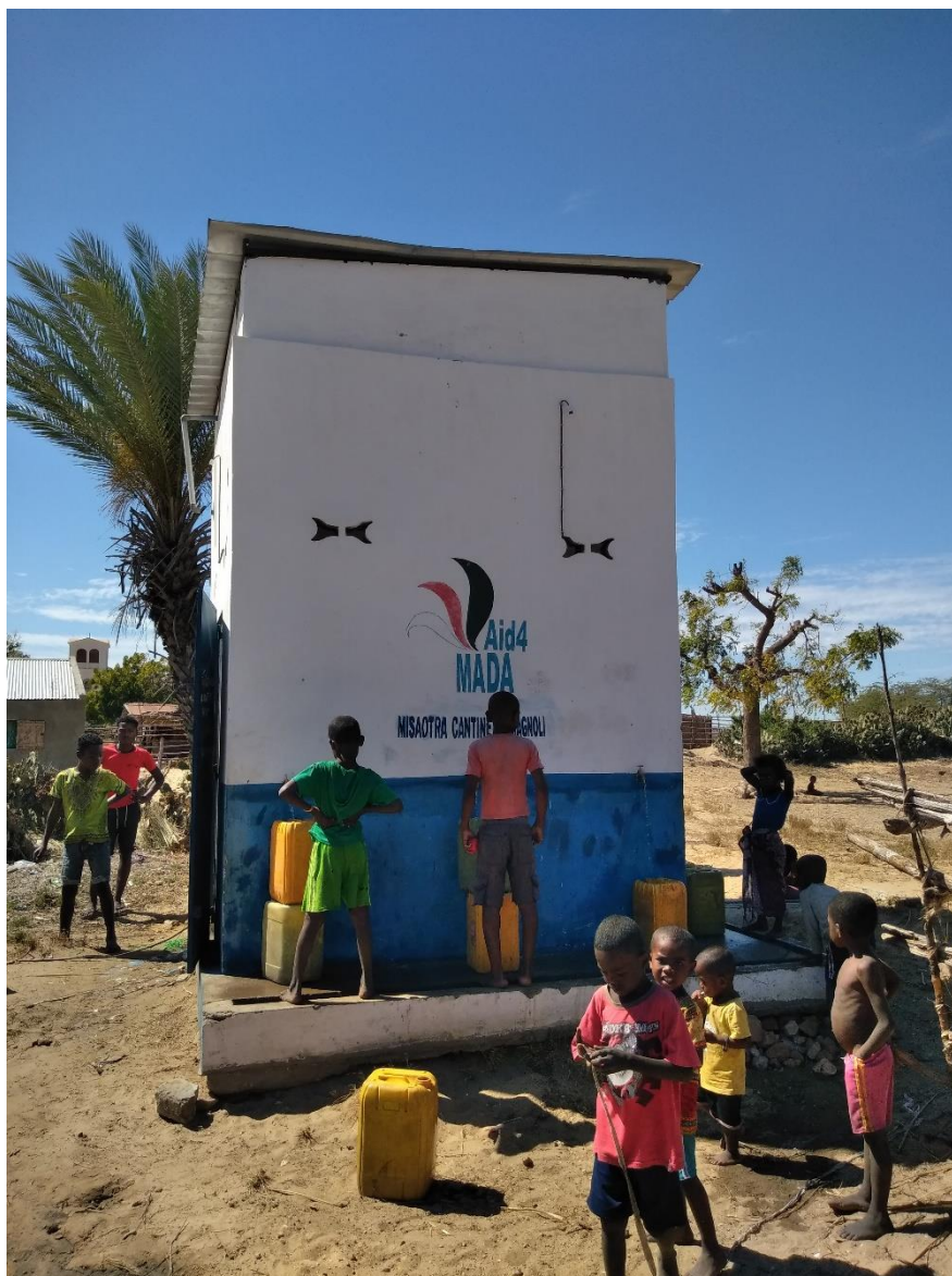
Imagine A-2. Project water system constructed in Andranomena village
