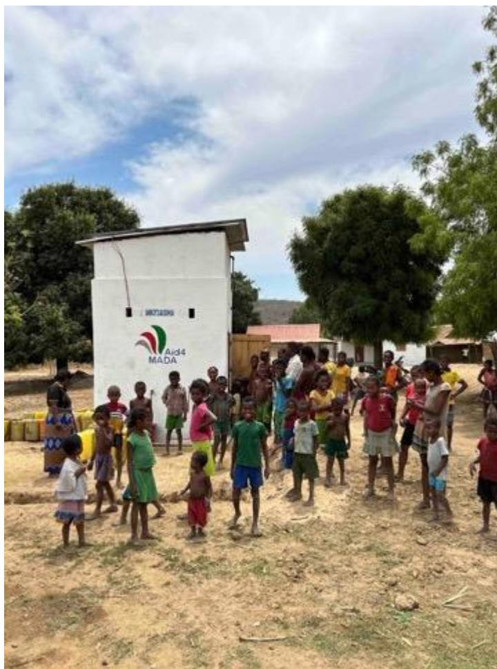
Imagines A-13. Project water system constructed in Ankotsahobihia village (GS10783)
