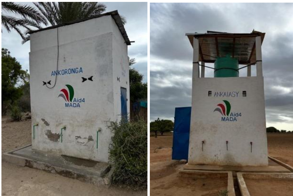
Imagines A-7, A-8. Project water systems constructed in Antobe and Ankoronga villages (GS10658)
