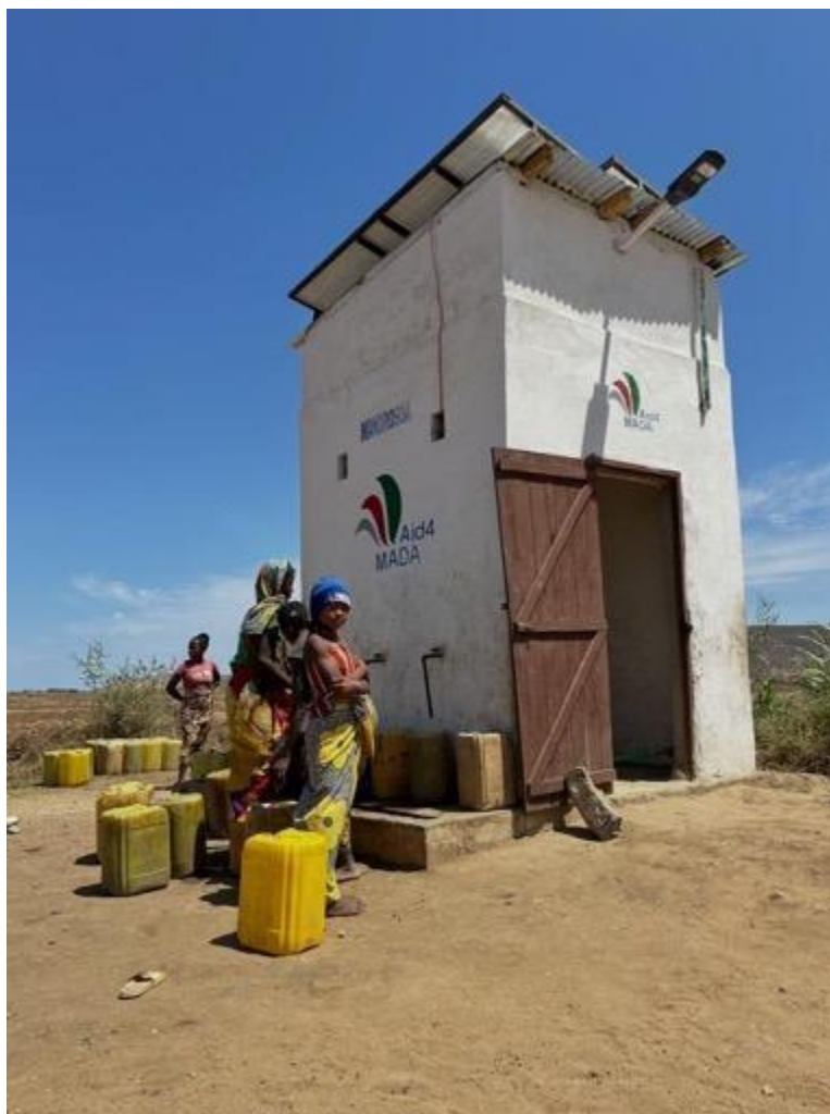
Imagines A-11. Project water system constructed in Mandrosoa village (GS10783)
