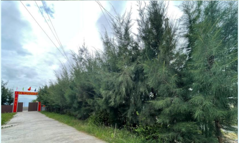
Trees at transformer station
