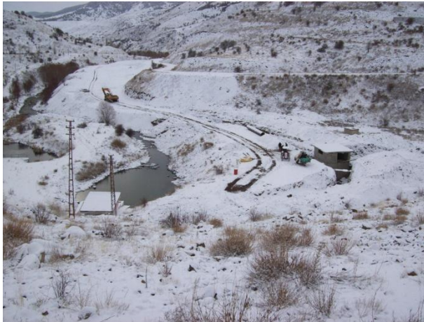
Figure.3. Penstock (Below Ground)
