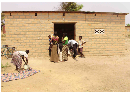
Plate 4: Household within project boundary
