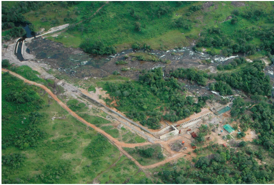
Plate 9: Plant site after Completion in April 2008.
